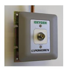
nameplate and the rough-in shall be a double O-ring which is serviceable without shutting off the gas service and is capable of supporting 10 pounds at 2" from the nameplate without leaking.
