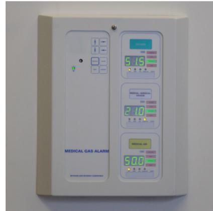
Area alarm shown is 3 gases – part #PX-DUXXOVA
