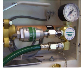
Dual port EZ Backfeed™ fitting with gauge, transducer, and backfeed hose attached to DISS gas specific demand valve shown above
